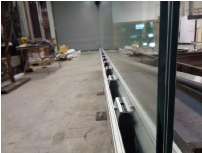
Photo No. 16 Support Rail with Bar Clamps Installed
